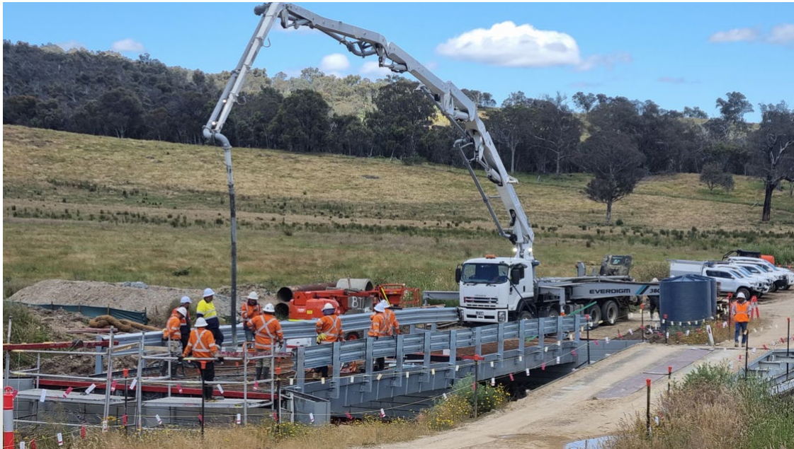
Works on Cooksvale Road Bridge
