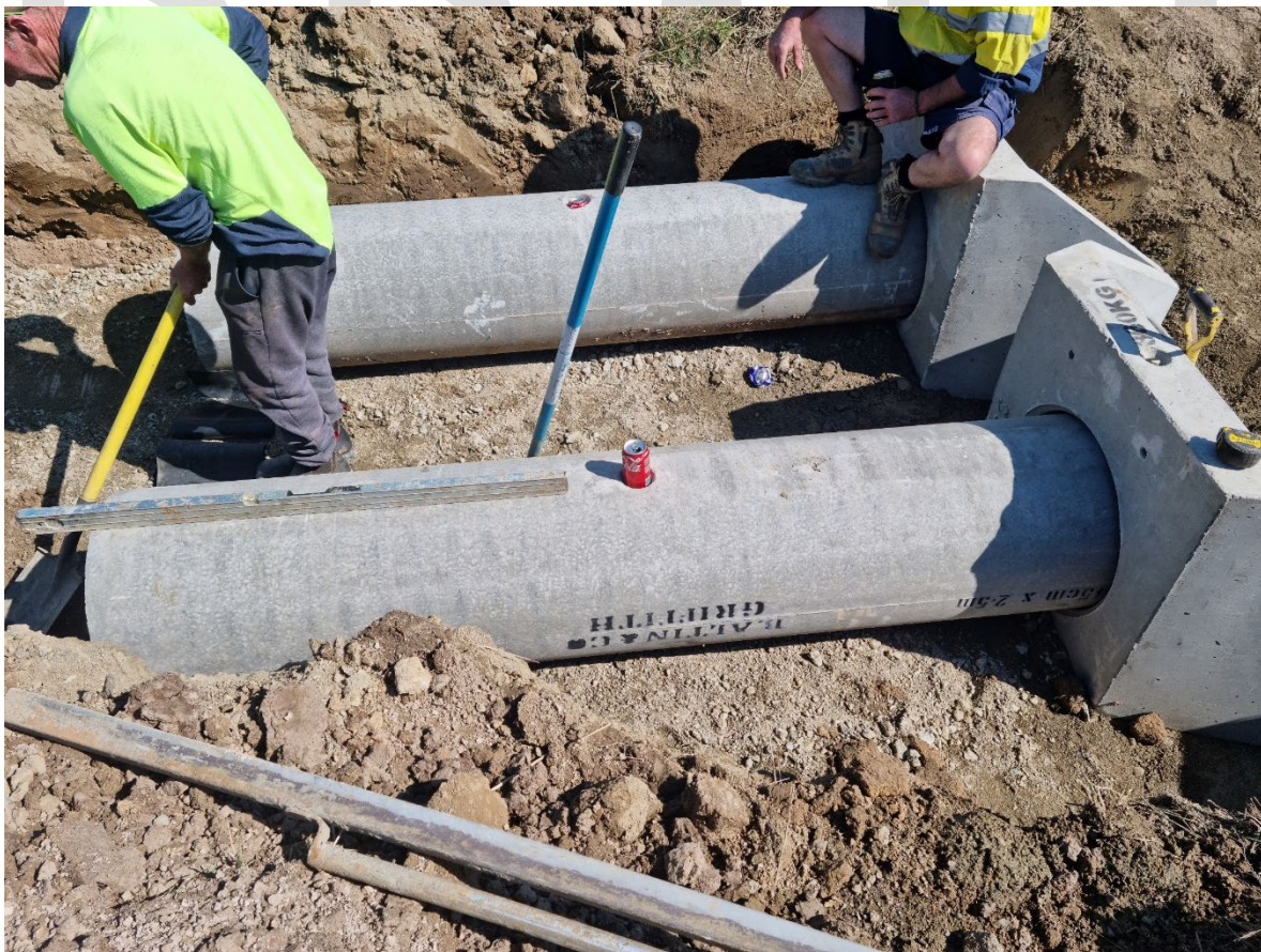
Pejar Road – Pipe removal and replacement
