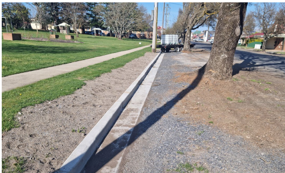
Kerb and Guttering works at Memorial Park in Crookwell
