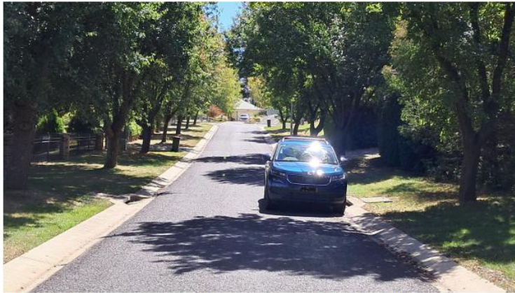
Photo 1: View north of Barry Place showing vehicle parked at kerb in front of No 12.
