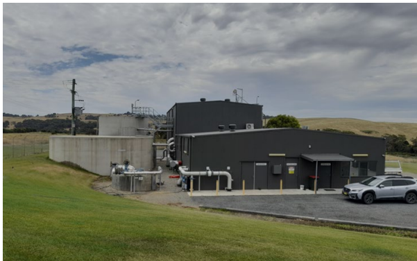
Crookwell Water Treatment Plant
