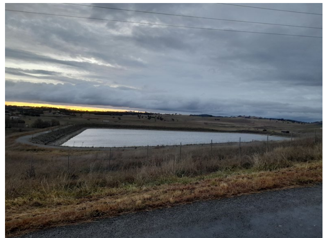
Gunning off River Water Storage Dam
