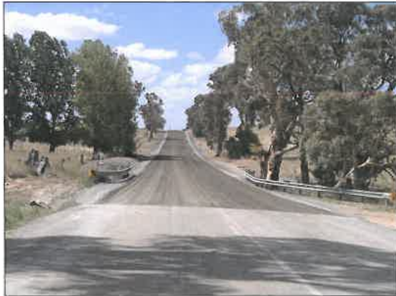
MR52 road reconstruction and bitumen resealing
