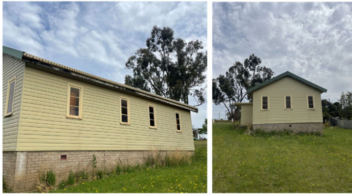
AN EXTRACT FROM THE PHOTOGRAPHS TAKEN BY LACHLAN BOLWELL. ABOVE: THE EAST + SOUTH ELEVATIONS, NOTE THE RELATIVELY RECENT TIMBER AND BRICK c1920. BELOW: THE UNDERFLOOR WITH CONCRETE STUMPS AND THE CEILING SPACE APPARENTLY WITH ASBESTOS LINING. SOURCE: LATERALS PLANNING.
