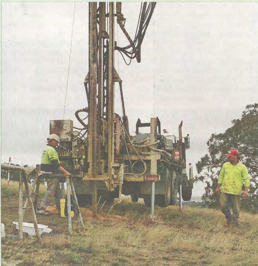
In February 2008, core samples were taken to establish geotechnical conditions for turbine foundations.
