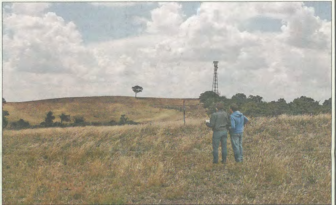
Contractors from the turbine supplier checking Turbine sites for crane and hardstand sitings.
