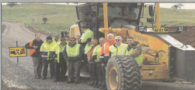
MR 52 is sealed! With only minor road work to be completed before its grand opening, scheduled for early in the new year, this vital road link between Gunning and Crookwell is now open for traffic
