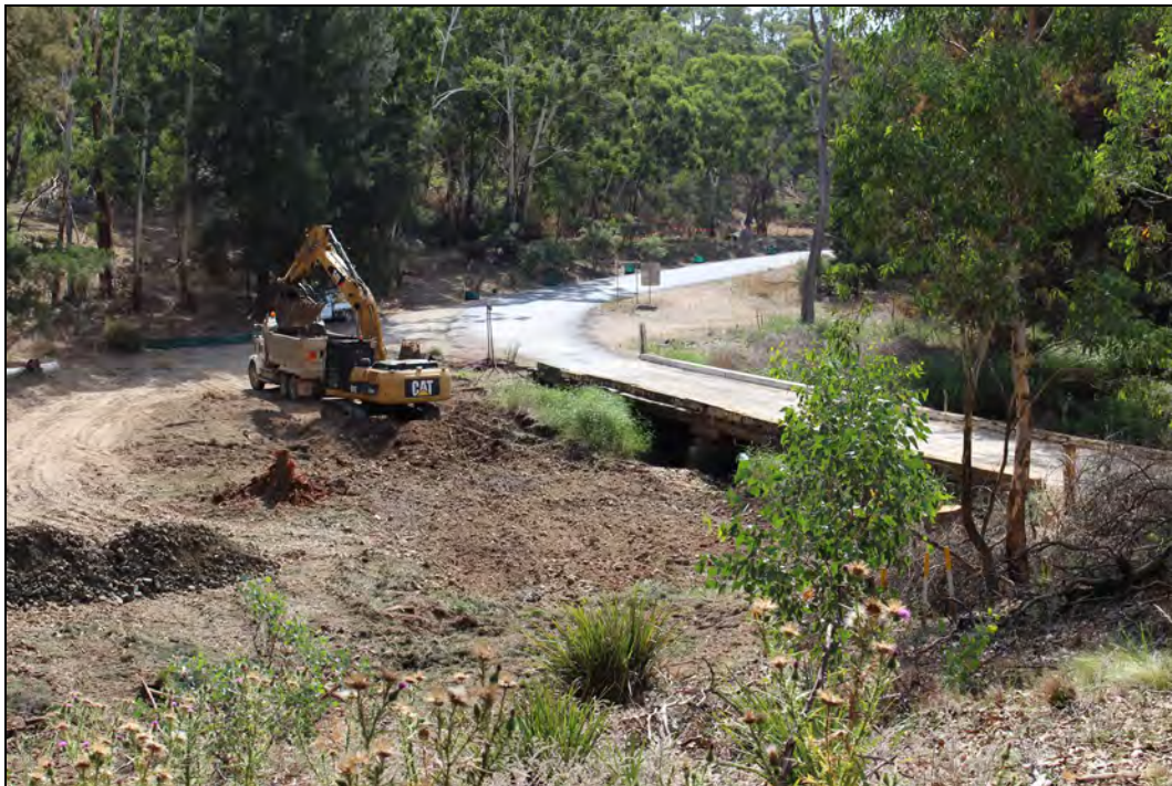
Commencement of the MR256 Oberon Road, Abercrombie River timber bridge replacement
