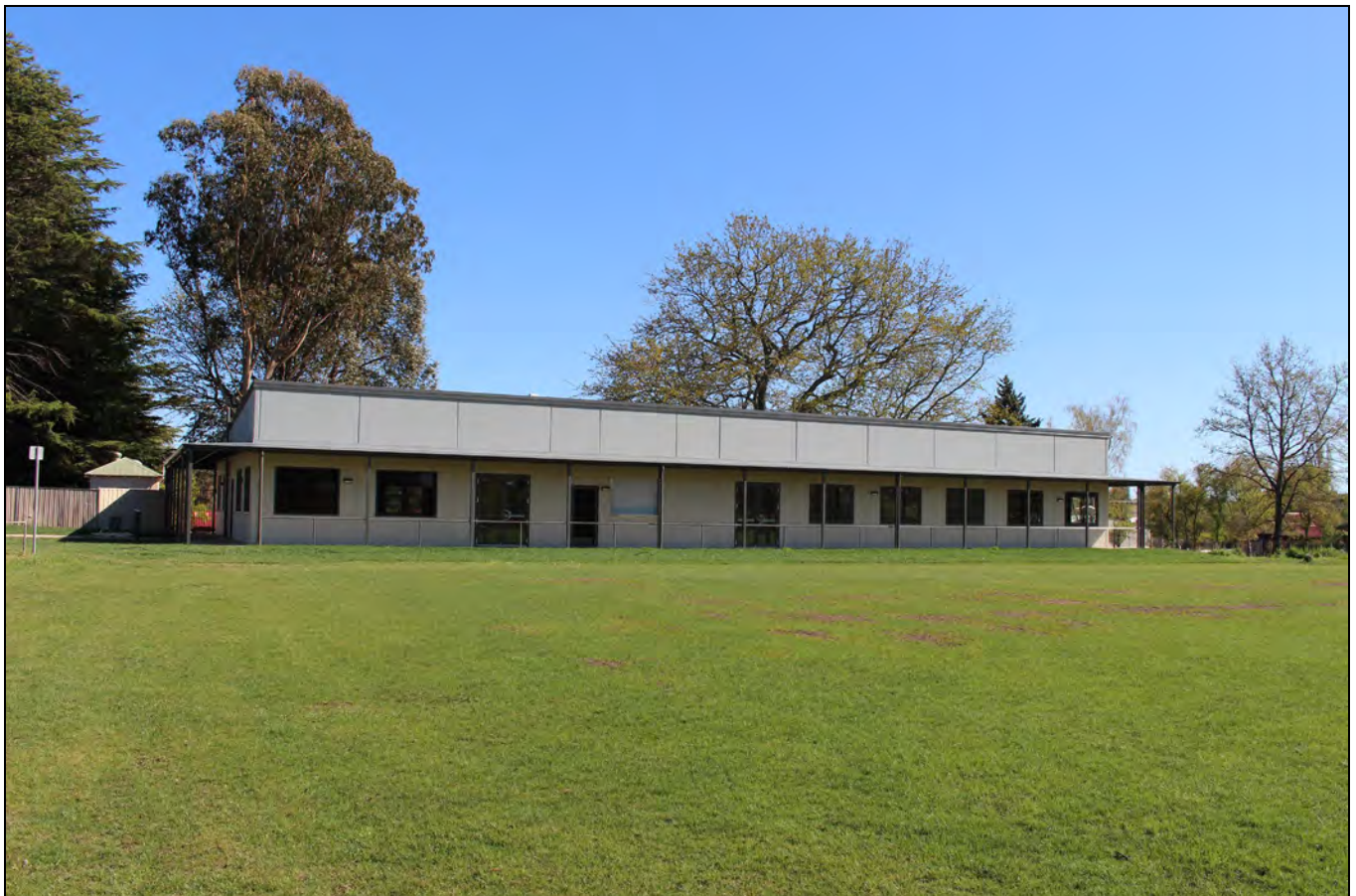
Crookwell Memorial Oval building construction project
