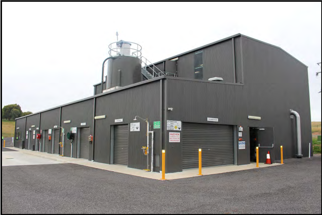
The Crookwell Water Treatment Plant commissioned in 2018
