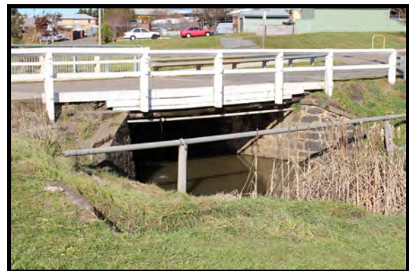
Kiamma Creek Bridge
