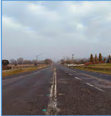
Figure 4a: Yass Street looking West from the intersection with Wombat Street
