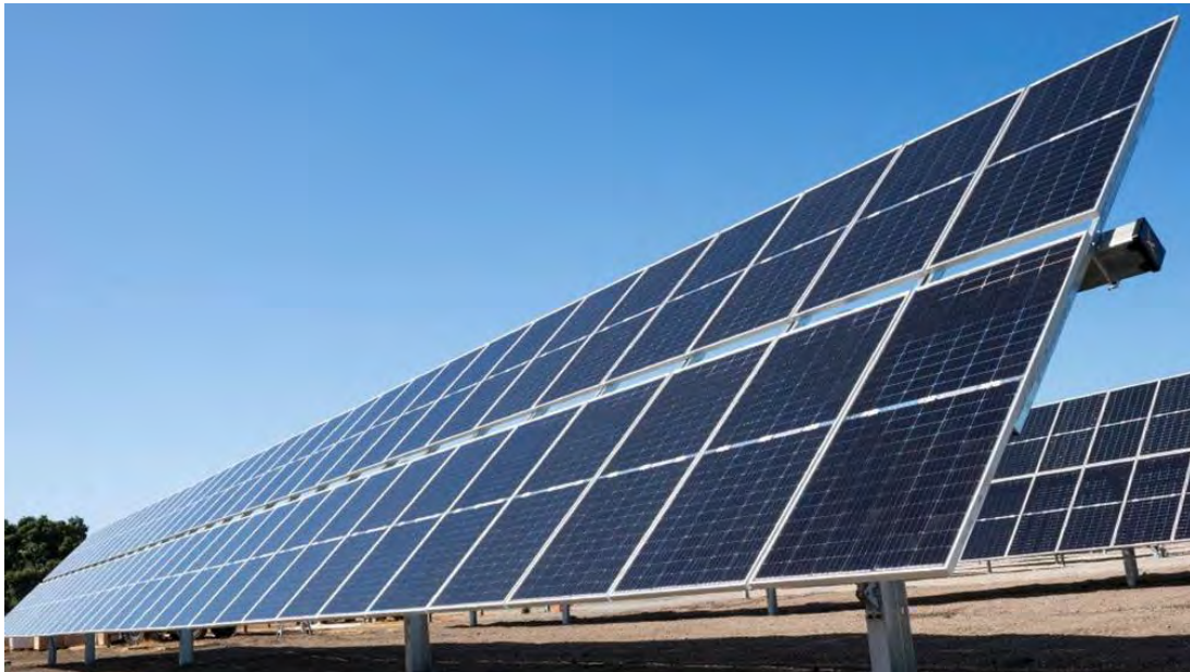
Photo 3.1 Example of PV Module Layout (2 in portrait or 2P configuration) (Nexttracker 2018)
