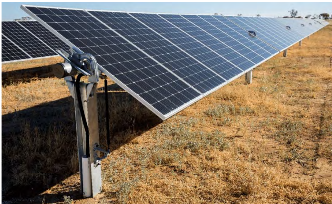
Photo 3.2 Example of a PV module layout (1 in portrait or 1P configuration) (Nextracker 2018)
