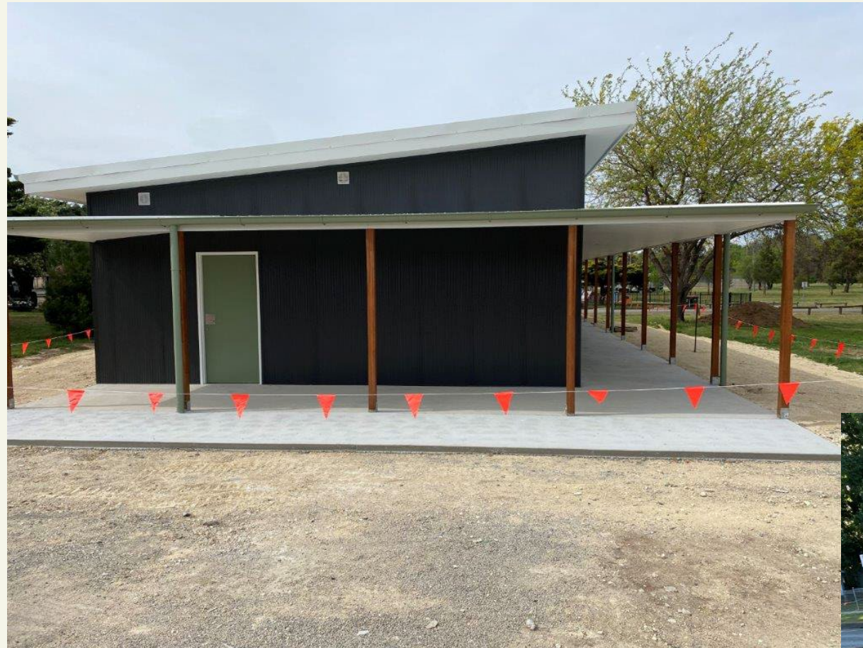
Gunning Electrical upgrades Showground amenities
