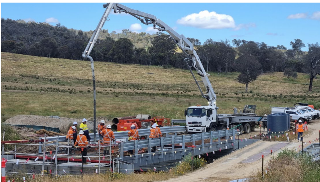
Cooksvale Road bridge construction
