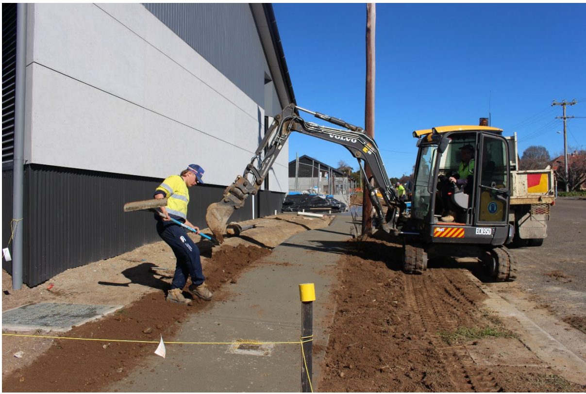
Footpath Upgrades, Crookwell
