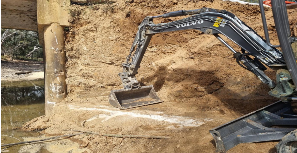
Works on Foggs Crossing Road
