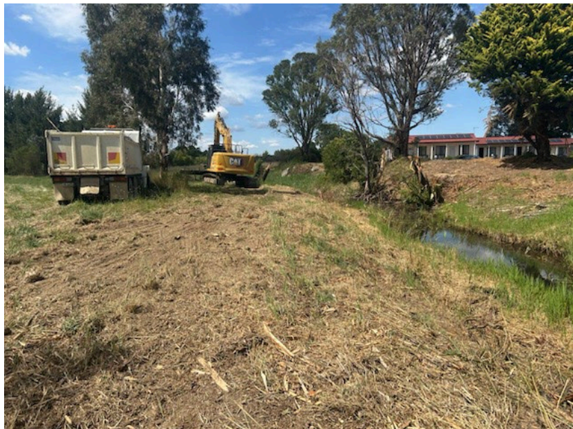
Works at Meadow Creek, Gunning
