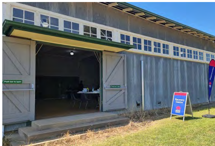
Gunning Shire Hall
