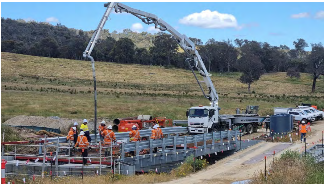
Cooksvale Road bridge construction
