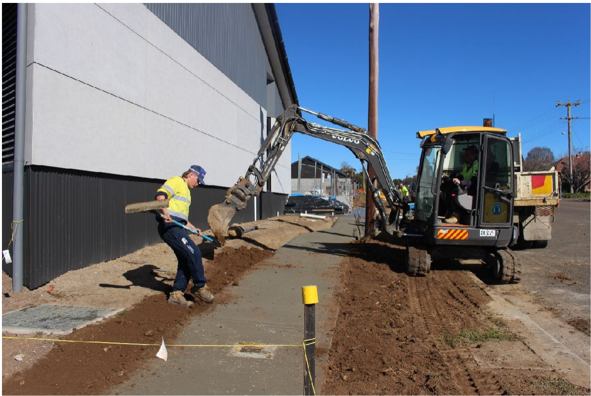
Footpath Upgrades, Crookwell
