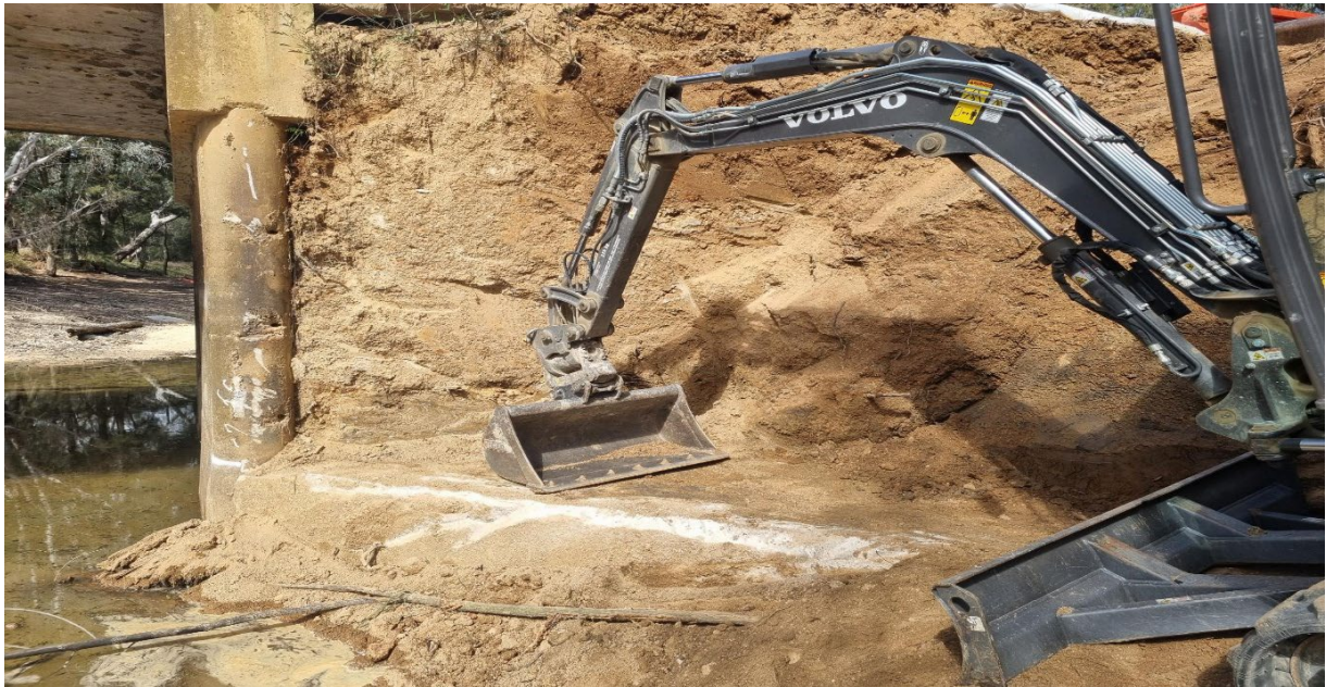
Works on Foggs Crossing Road
