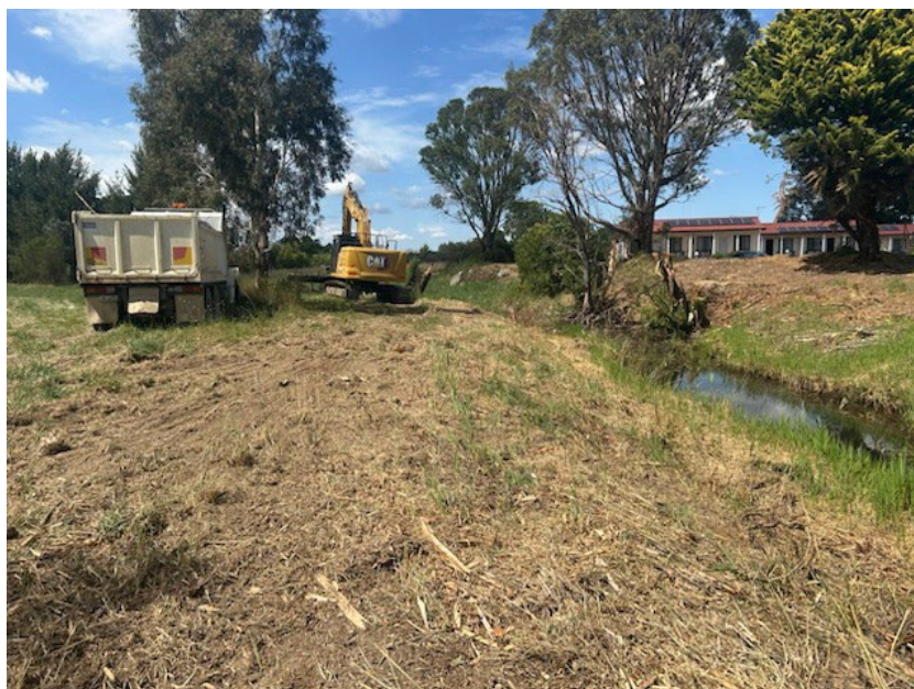
Works at Meadow Creek, Gunning
